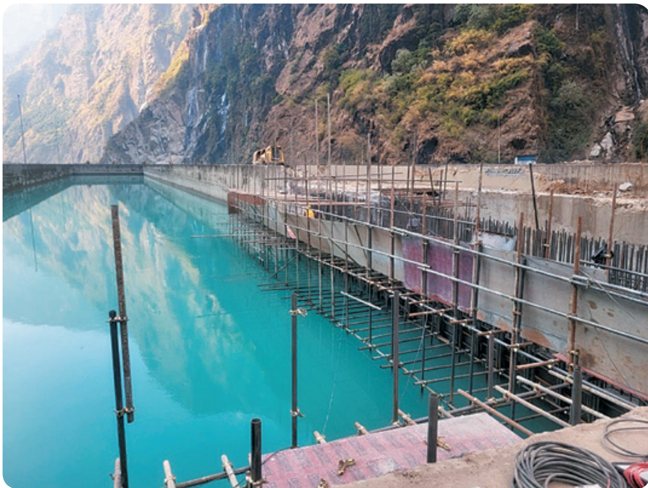
Left Settling Basin Operation after Repair Works
