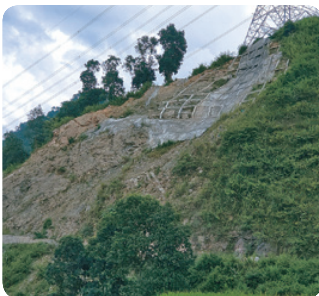
Completed Design and Supersision of Tower Protection works for T15, Khimpti –Dhalke 220 kV TL
