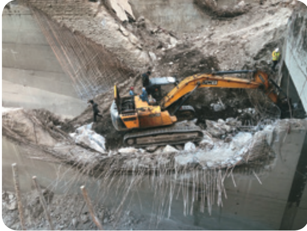
Damage on Baffle and Central Wall of Left Settling Basin
