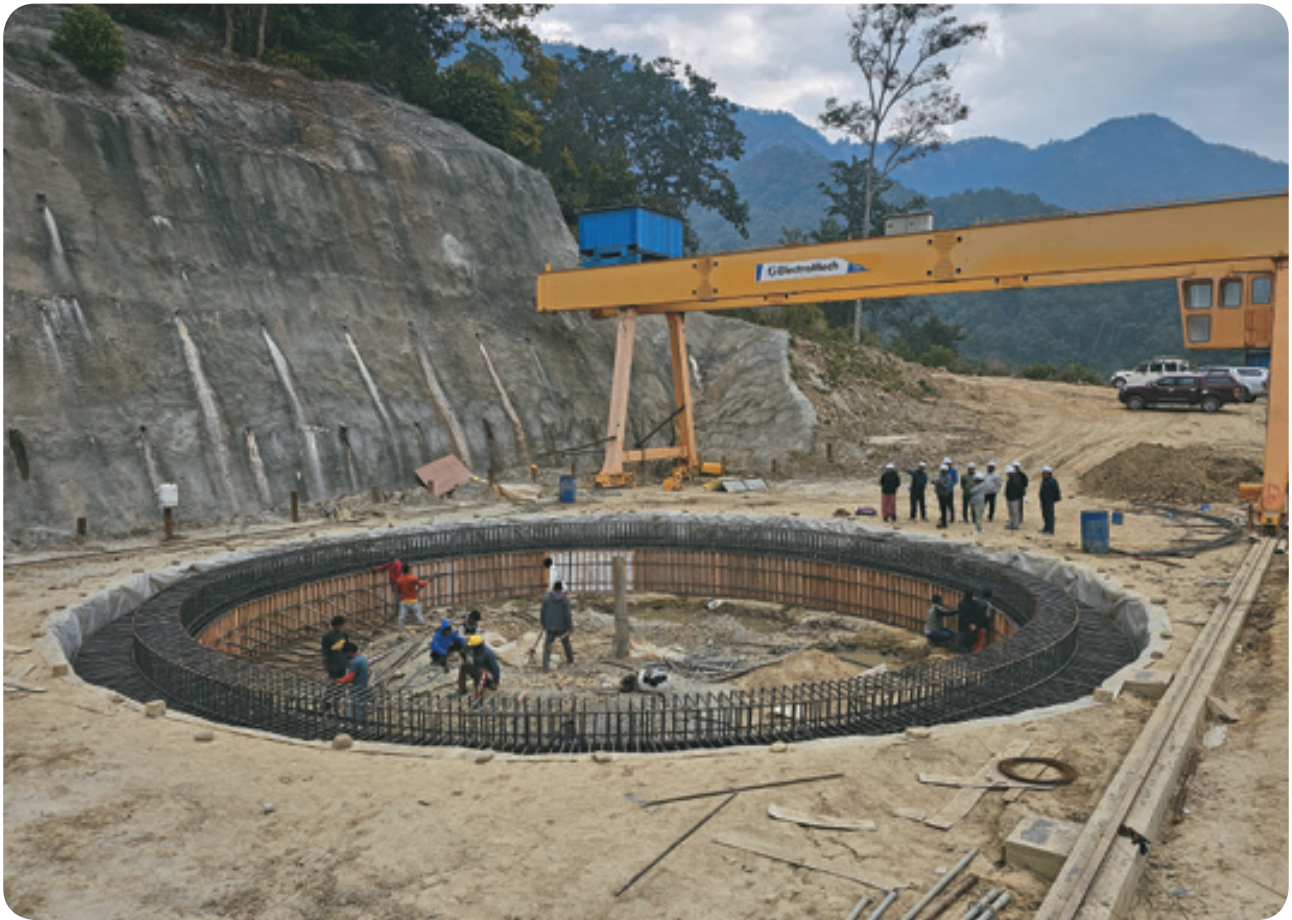
Construction of Colar Beam for Surge Shaft
