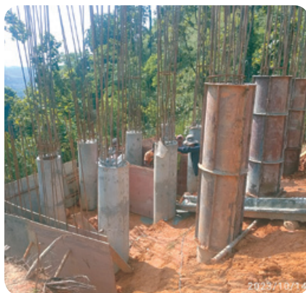
Construction of Pile Foundation for 100 m Tall Tower LL5 Hetauda–Bharatpur-Bardaghat 220 kV TL
