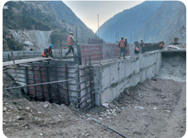
Repaired Central Wall of Settling Basin to Top Level
