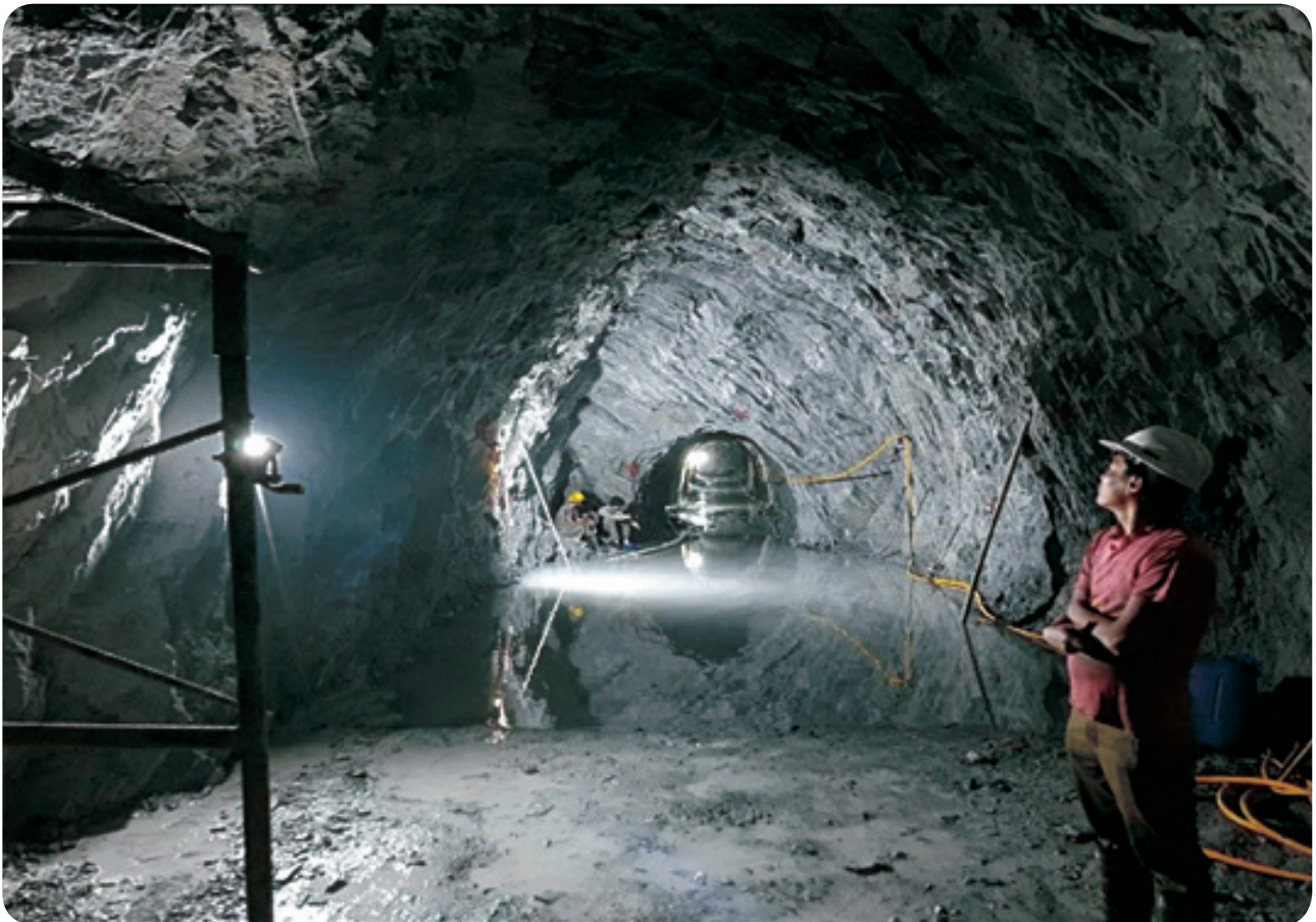
Test Tunnel in Powerhouse Cavern of Jagdulla PROR HEP
