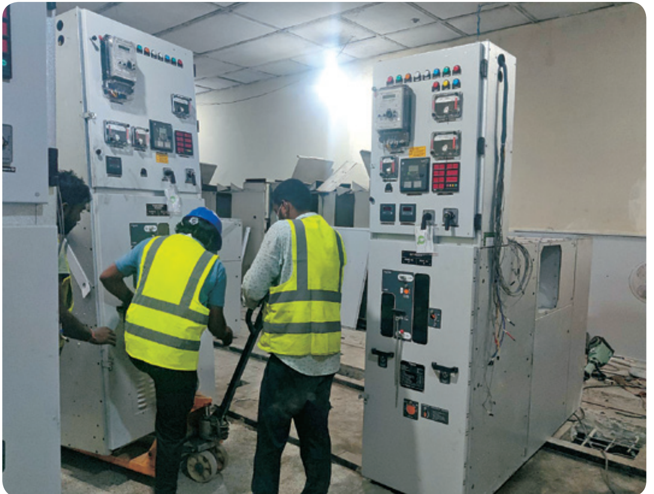
Installation of 6.6 kV Switchgear
