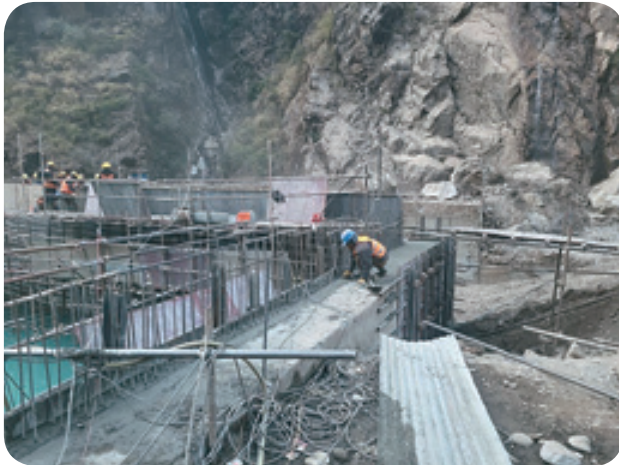
Repair Works on the Headwall of Box Culvert
