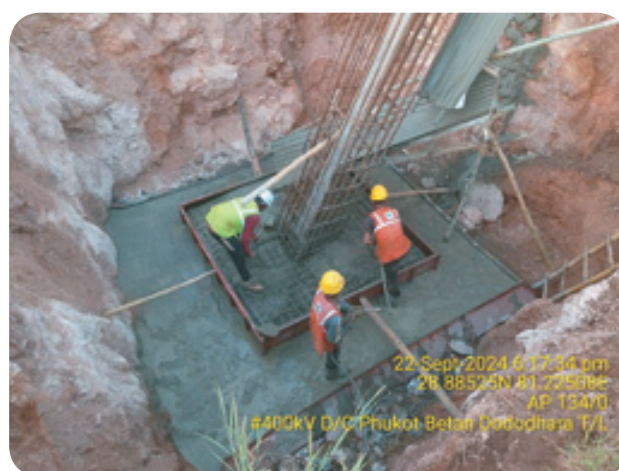
Casting of Tower Foundation for Tower Type DB
