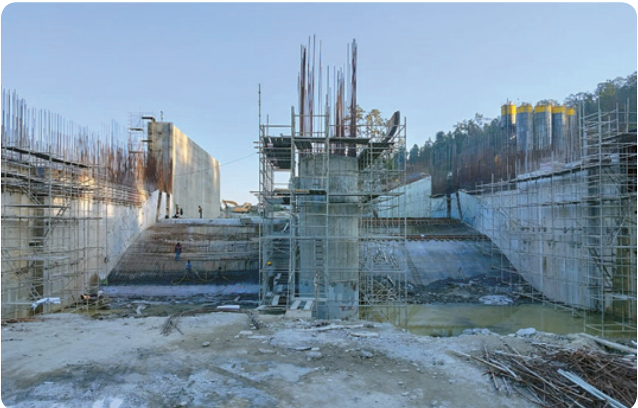
BBDMP Close View of Under Sluice in Head Works
