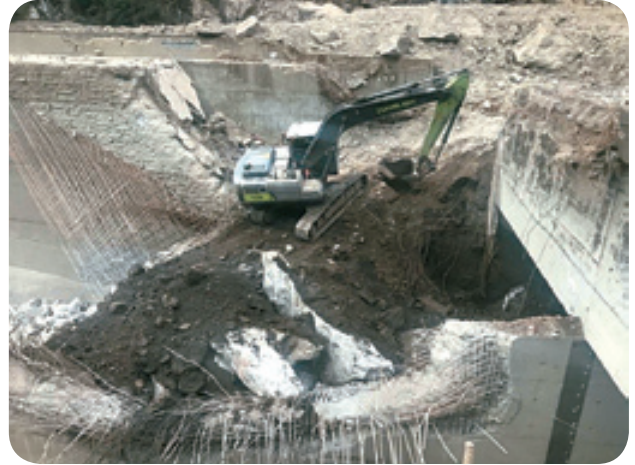
Damage on Left Settling Basin and Headwall of Box Culvert
